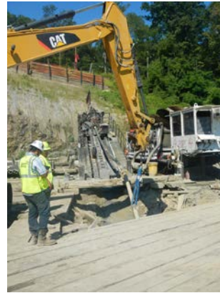
Title: 08-28-16 MP 3.00 deformation in drill stem at rig - Hudson River HDD west during installation.
