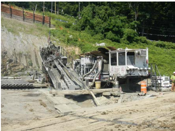
Title: 08-29-16 MP 3.00 deformation in drill stem at rig - Hudson River HDD west during installation.
