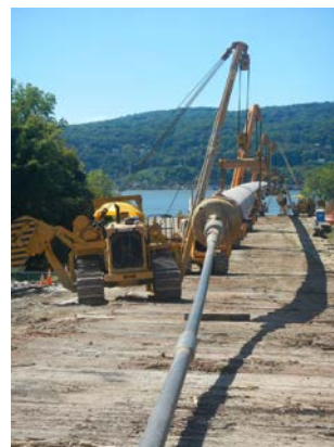
Title: 08-29-16 MP 4.08 pipe segments suspended drill stem at Hudson River HDD east side.
