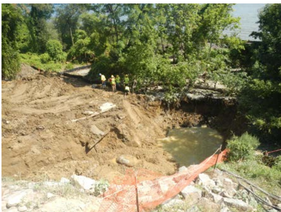
Title: 08-29-16 MP 3.01 unapproved ground disturbance in wetland A14-SPLR- W100 at Hudson River HDD west.
