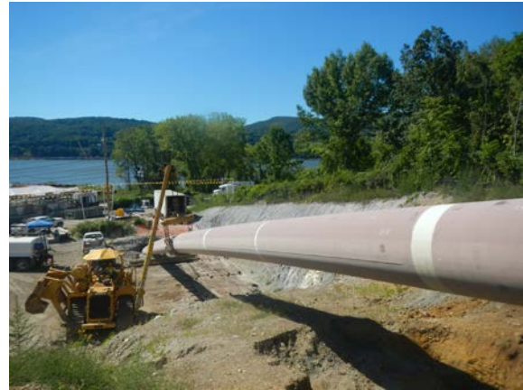
Title: 08-29-16 MP 3.93 suspended pipe at Hudson River HDD east side installation.
