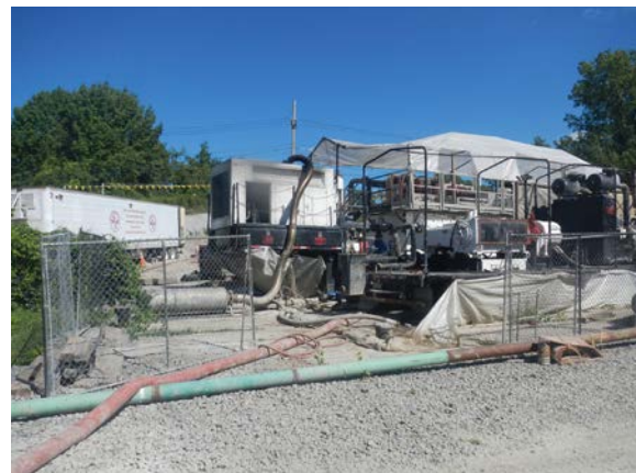
Title: 08-29-16 MP 3.91 mud recycling rig in secondary containment at Hudson River HDD east.
