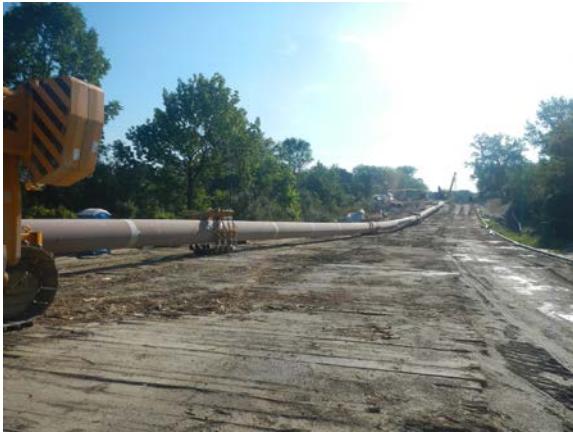
Title: 08-28-16 MP 4.02 inactive pull-back at Hudson River HDD east side.
