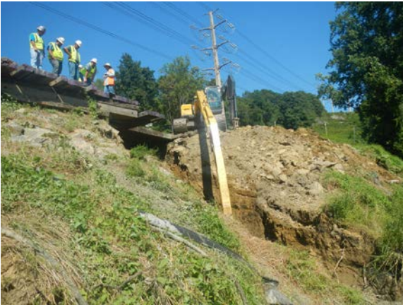
Title: 08-28-16 MP 2.99 excavation over HDD centerline to wetland A14-SPLR- W100 boundary at Hudson River HDD west.
