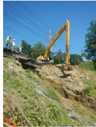
Title: 08-28-16 MP 2.99 excavation over HDD centerline to wetland A14-SPLR- W100 boundary at Hudson River HDD west.
