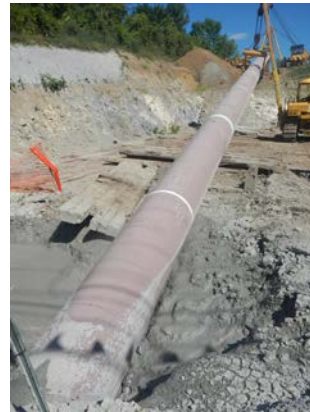
Title: 08-29-16 MP 3.91 insertion point for Hudson River HDD east installation.
