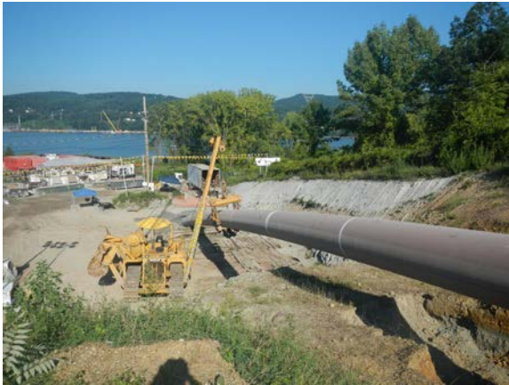
Title: 08-28-16 MP 3.93 inactive pull-back at Hudson River HDD east side.
